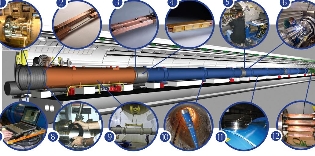
18 000 electrical Quality Assurance tests 10170 leak tightness tests
